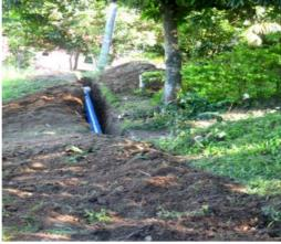
Pipe laying of 6" uPVC Pipe and installation of other appurtenances at VDC, Brgy. La Mesa
