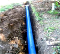
Excavation of trenches and laying of pipes at Indigo Bay Subd. Ph2, Bagong Kalsada
