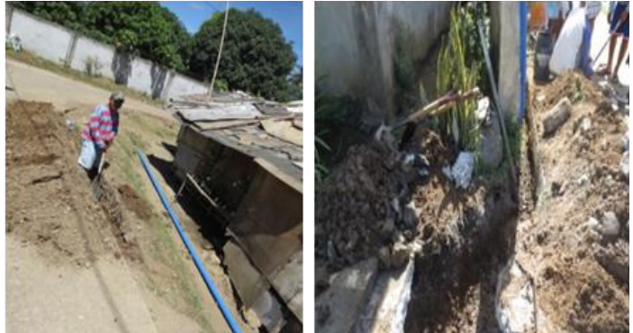
Rehabilitation of waterlines along Brgy. Bubuyan.
