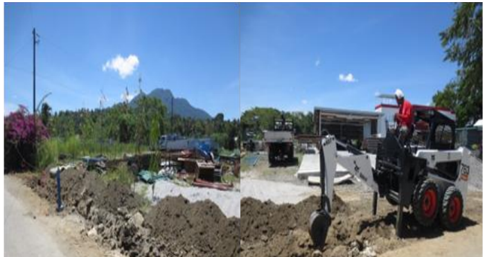
Expansion of waterlines along Brgy. Maunong.
