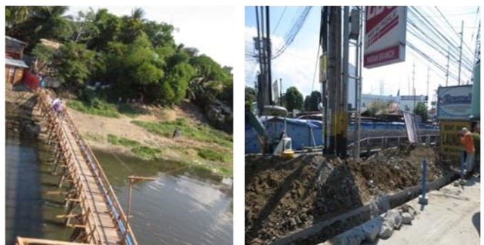
Temporary Relocation of waterline along Brgy. Bañadero, Brgy. Parian and San Cristobal bridge.
