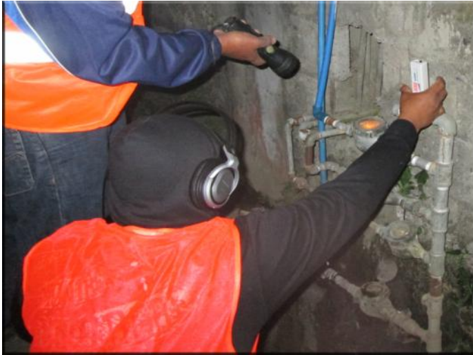
WSMD Field Staff conducting leak detection at Villa de Calamba using the newly acquired gadget that will help reduce non-revenue water and improve water pressure.
