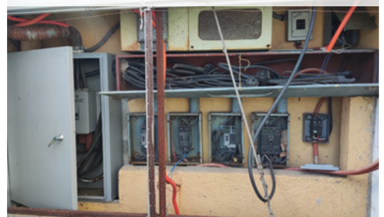
Electrical Rehabilitation Project
